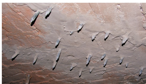
Vaulted ceiling underneath the Library of Commerce with installed injection packers
